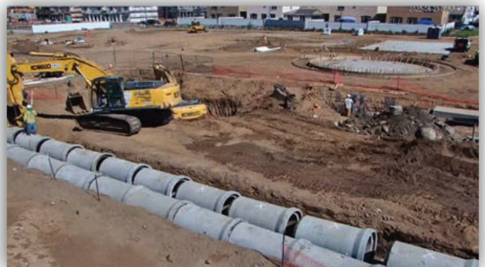
Construction of the Orchard Run Lift Station.
